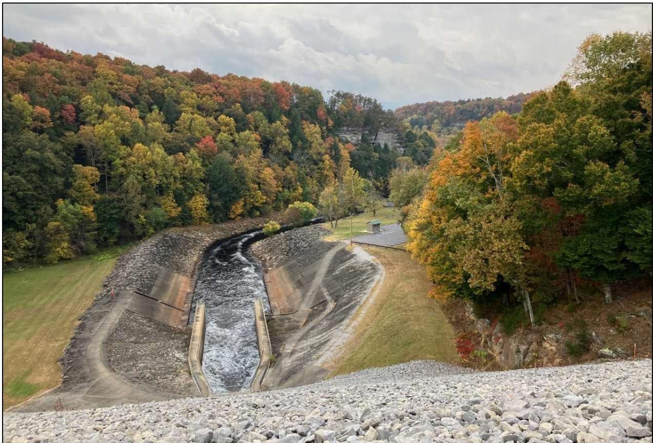
Nolin River, Nolin River Dam and outflow (USACE photo)
